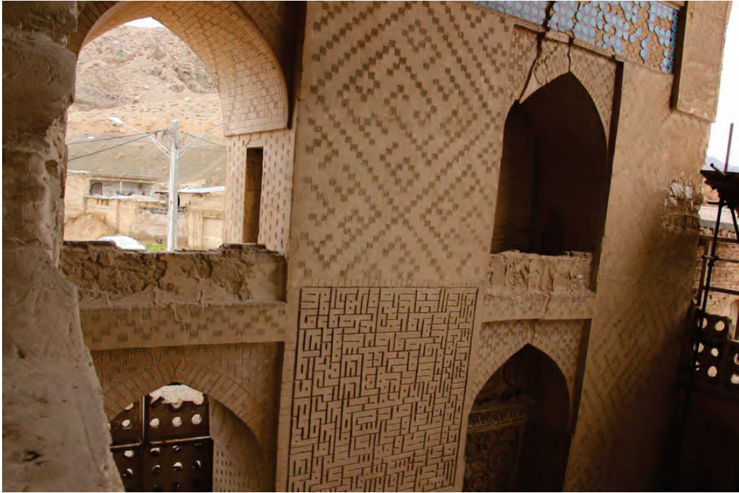
Img. 16: Adhesion mortar, which corresponds in dimensions to the New York and Berlin tiles with phoenix images and Qur'anic quotations and suggests their original location in the Pir-i Bakran mausoleum. (Grbanovic 2018)
