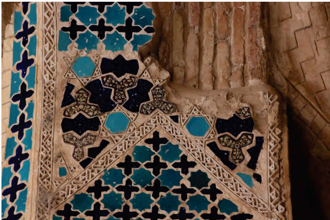
Img. 7: Luster tiles of the Pir-i Bakran mausoleum (first decorative stage) were likely reapplied on its architectural surfaces during restoration interventions. The tiles are currently located in the intrados of the ivan's ceiling. (Grbanovic 2014)
