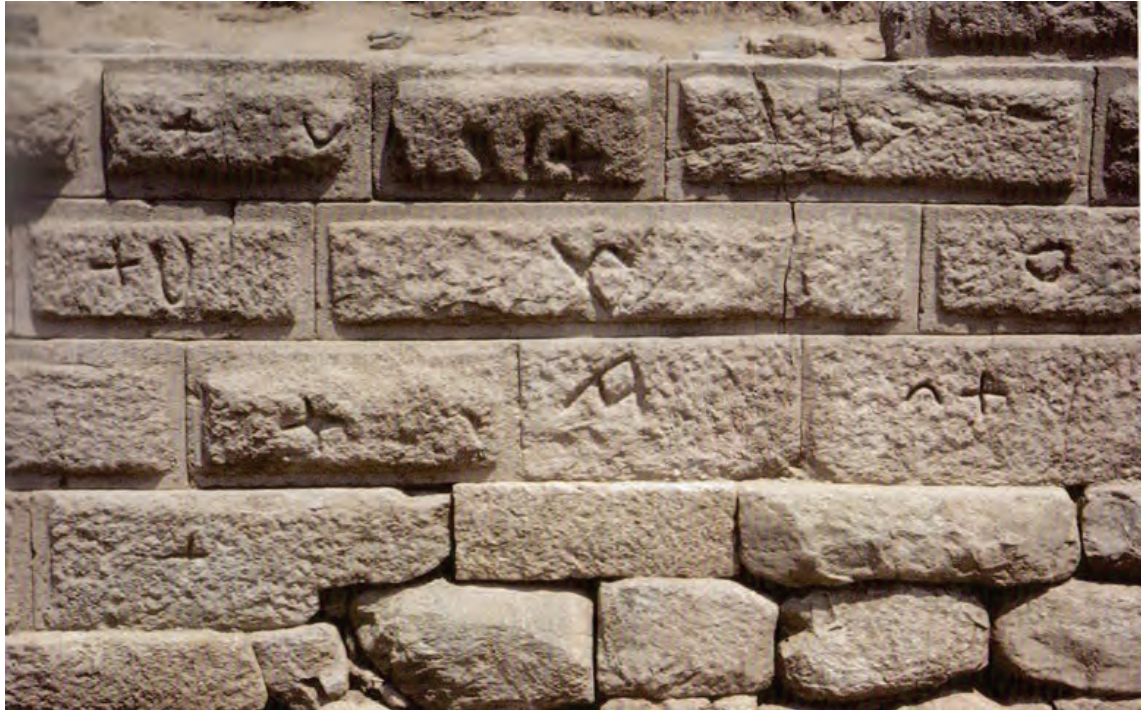
Fig 4. Ashlar masonry with mason's marks from gate of Lydian fortifications at Sardis (after Cahill 2010)
